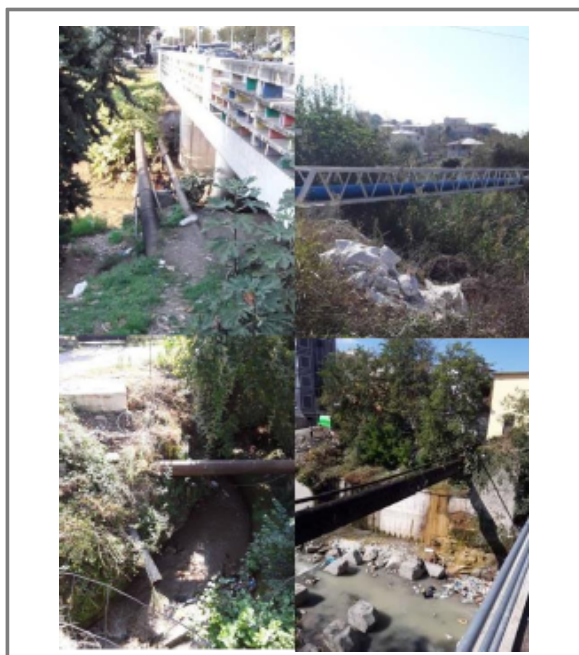
“Aqueduct” (08-06-L, A-01)
